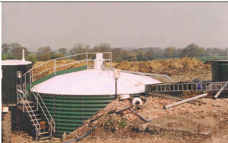
Photograph of digester under construction in 1992
